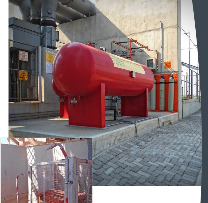
A Protect-o-Burn vessel is filled once with potable water, and then it is disconnected from permanent water supplies.
